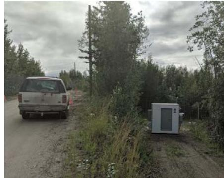
Blower enclosure building for air sparge system.
