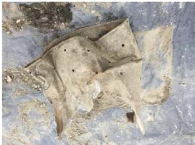
Drywell constructed of perforated 55-gallon drum
